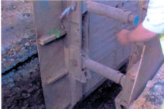
Figure 8: Trench Box Being Used to Prevent Collapse of Excavation
