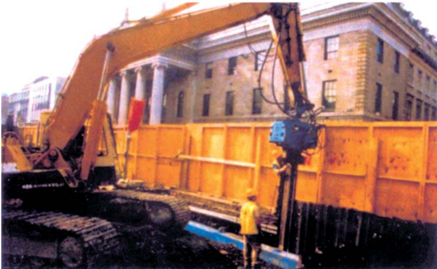
Figure 13: Installation of Excavation Supports Under Supervision
