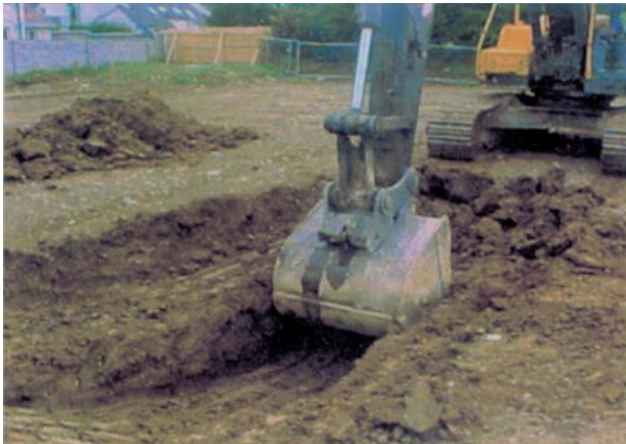
Figure 10: Spoil being Piled Away from Edge of Excavation
