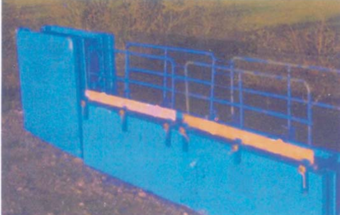
Figure 9: Trench Box with Handrails and Toe-boards
