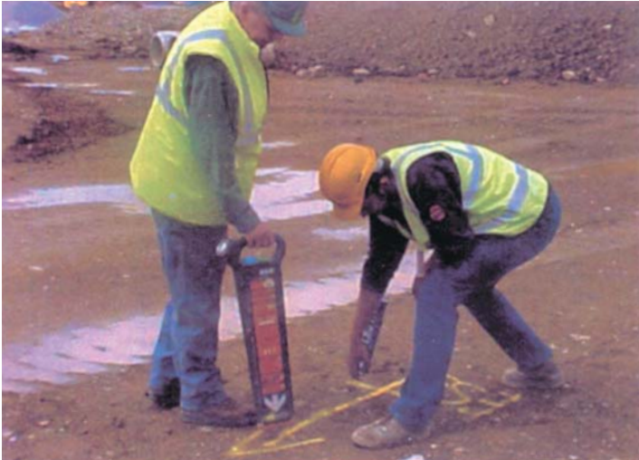
Figure 3: Operators on Site Locate Underground Services Prior to Excavating
